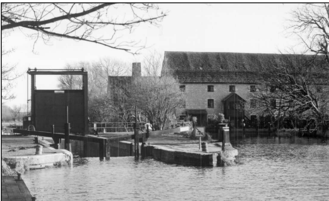
Fig 24g. Water Newton Lock, built during the upgrading of the 1930s, now with a motorised guillotine gate.
