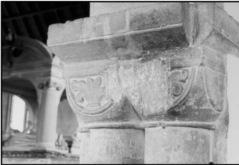
Fig 15c. Chancel Arch - the shafts with their cushion capitals are not later than 1120.
