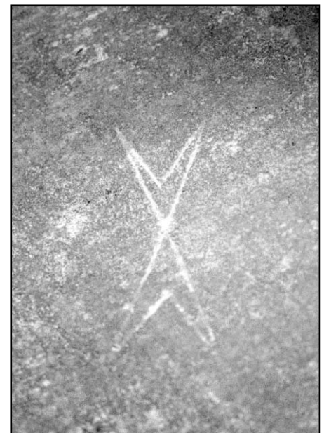
Fig 15i. Masons' Marks: these marks can be found in a number of places, including the balustrade, and appear to be associated with 17th century work in the North aisle. (Photo: NADFAS)
