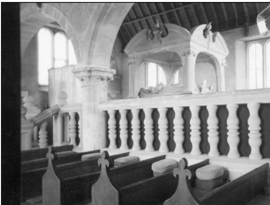
Fig 15h. The Dove Monument: the North aisle was elevated and rebuilt to accommodate the memorial. There are 14 lead coffins in the vault below.
